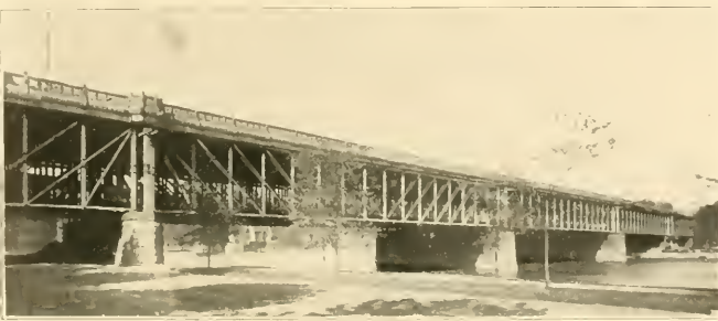
HIRARD AVENUE BRIDGE Fairmount Park
